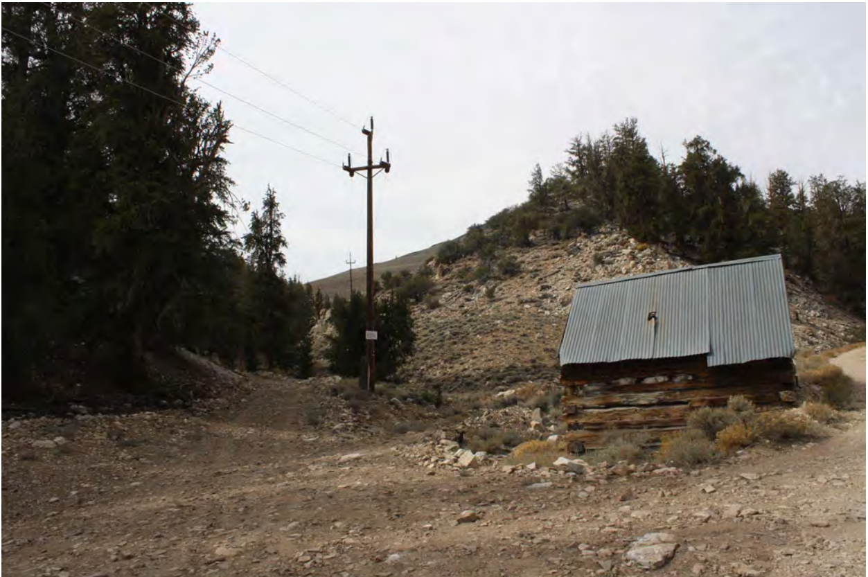
19. Wyman Creek Road at historic cabin looking west
