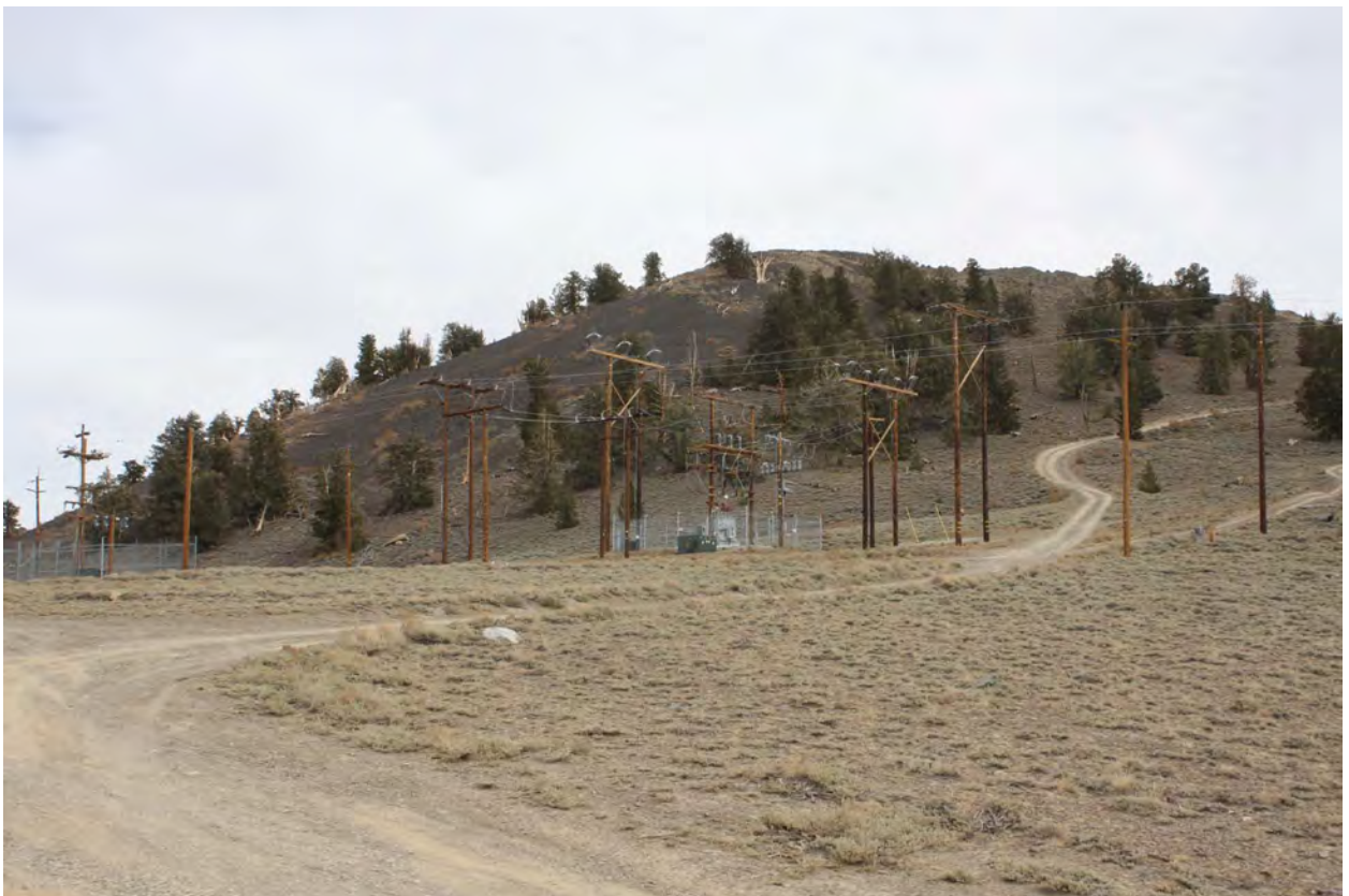
16. Silver Canyon Road near White Mountain Substation looking northeast
