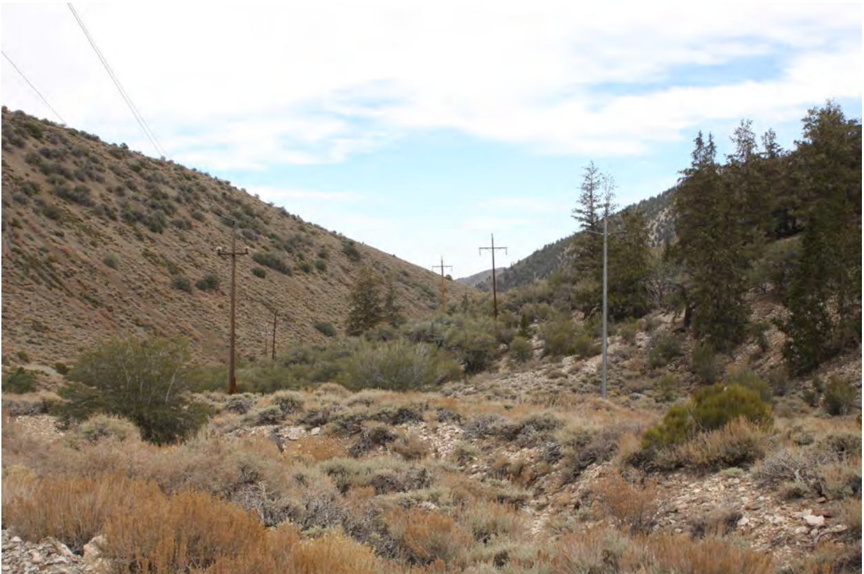
20. Wyman Creek Road in upper canyon looking east
