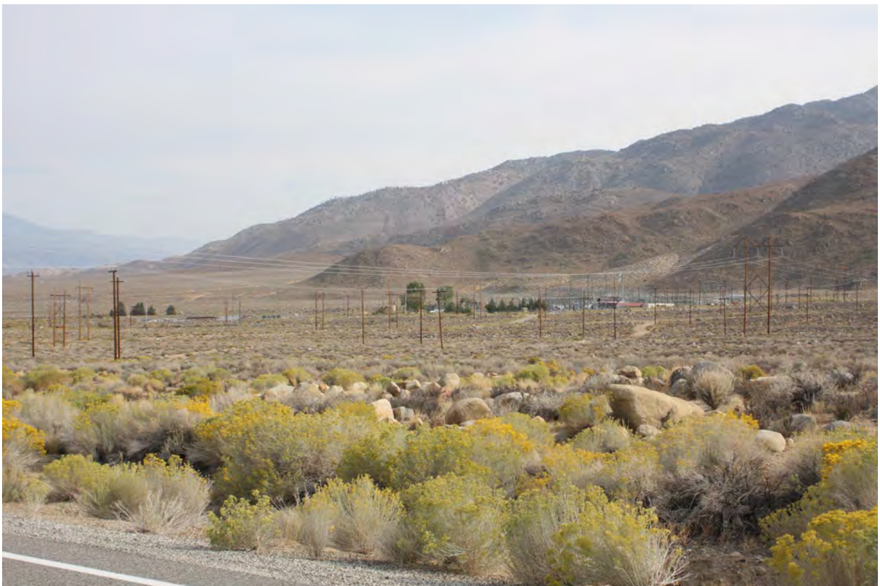
2. SR-168 looking southeast towards Control Substation
