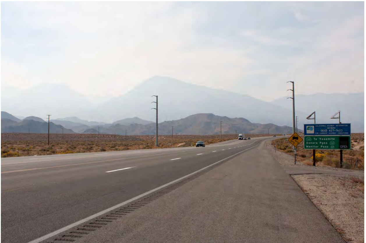
5. US 395 looking west
